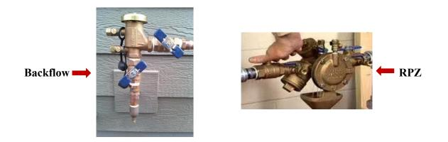
This new code states that homeowners are required to have this piece of equipment tested yearly by a licensed and certified backflow tester and filed with the municipality. The homeowner and tester are required to keep record of these tests.
